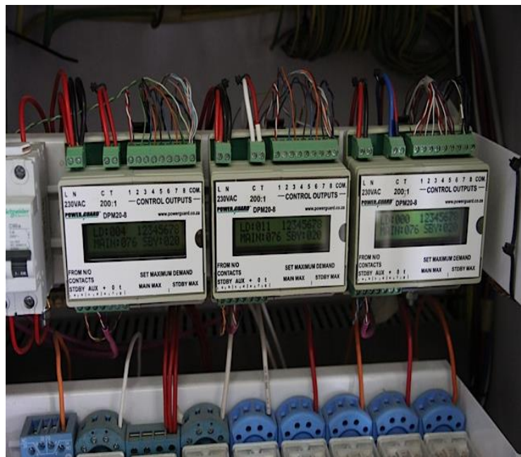
Figure 1: Arrangement of three 8-channel peak demand controllers
