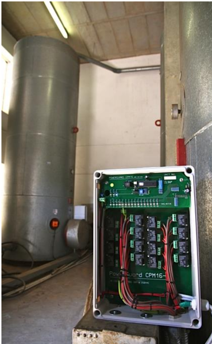
Figure 4: 200 kVA boiler array controlled by 16-channel units at a Johannesburg hotel.
